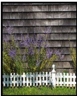
An increasingly popular siding is cement board products and they come in the form of panels, planks and even shingles. They are virtually maintenance free; they do need to be cleaned with the hose, a mild cleaner and some elbow grease from time to time – **again no power washers please!**
